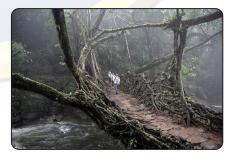
A living root bridge is like a suspension bridge formed by guiding the pliable roots of the rubber fig tree (Ficus elastica) across a stream or river and allowing the roots to grow and strengthen over time.
